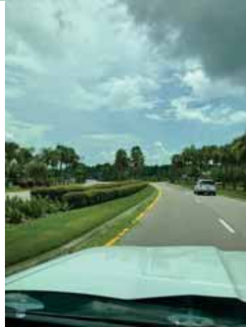
South Branch Blvd Center Medians.
