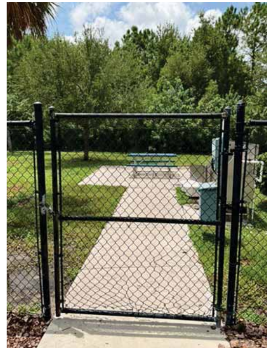
Adding a spring hinge to keep the gate closed & Patch Fence.
